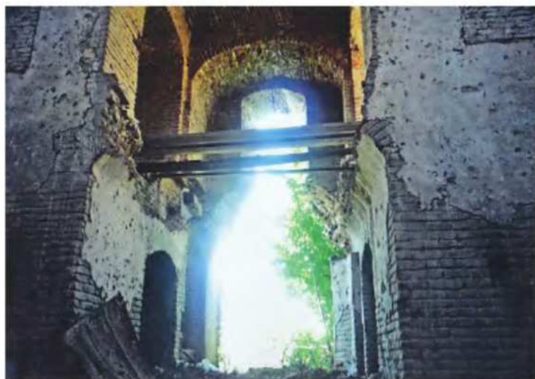
Fig. 4. The view of the two-story auxiliary rooms
