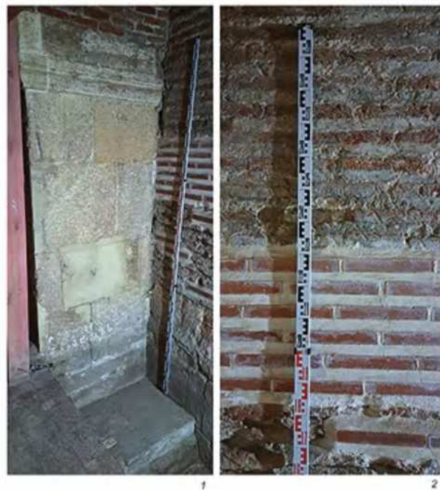
Fig. 6. Derbent. Juma Mosque. Interior. Eastern wall. Adjacency of the pilaster to the wall (1) and the nature of the brickwork (2)
