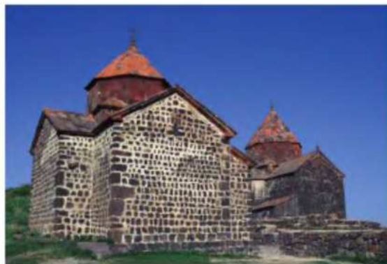
Fig. 18. Pay attention to the masonry of the church walls on the right and left!
