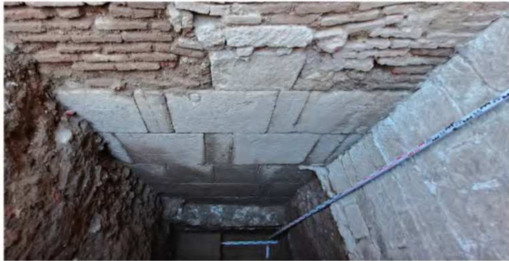
Fig. 2. Derbent. Juma Mosque. Southern wall. Pit 46. Brick and stone Sassanid masonry of the outer façade of the southern wall of the mosque. View from the SSE (South-South-East)
